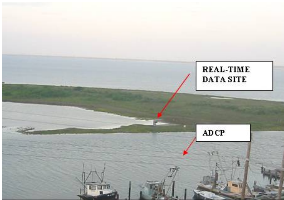
Figure 12. View from the JFK Causeway GIWW bridge of location of the data controller/logger/telemetry site and the bottom-mounted ADCP. A double armored cable connects the ADCP to the shore site.
